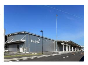
Peach Aviation requested that Terminal 2 have a simplified design in order to minimize operating costs. The terminal is a single-story building, thus eliminating the cost of elevators. Passageways to aircraft have no air conditioning. The terminal also has no boarding bridges, having 4 domestic, 3 swing, 2 international boarding gate. In case of rain, passengers are lent umbrellas to use as they walk to the aircraft.
